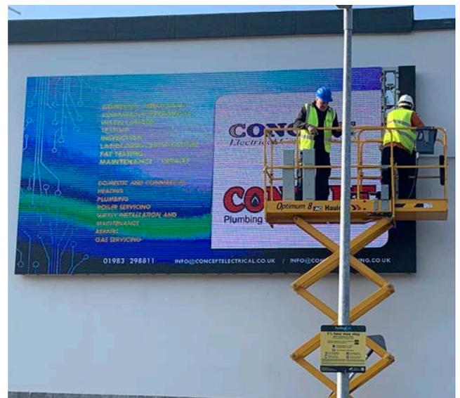
Our installation team managed the install, working alongside a local partner. The lightweight LED cabinet structure, as well as the magnetic modules and positioning pins, ensured a smooth installation.
